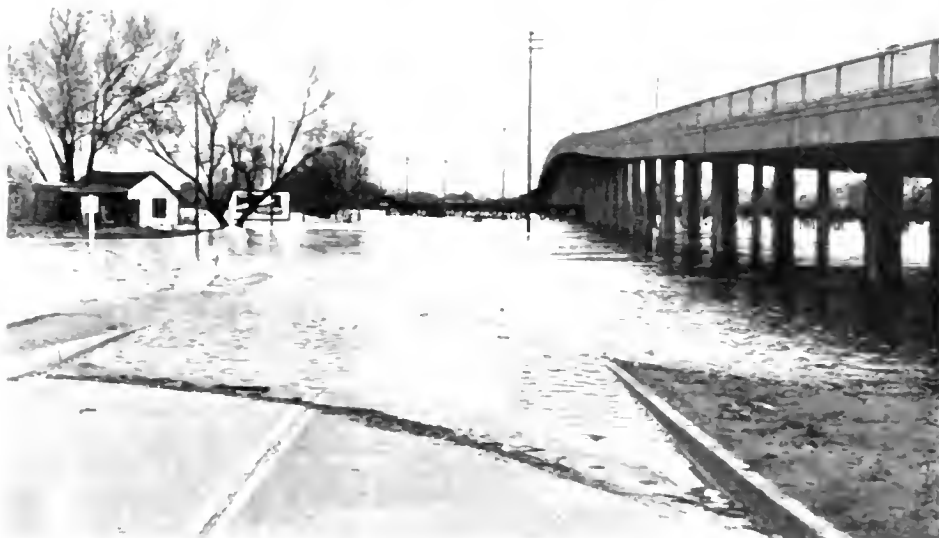
Viaduct 50 feet above ground level, crosses channel and two railroads
